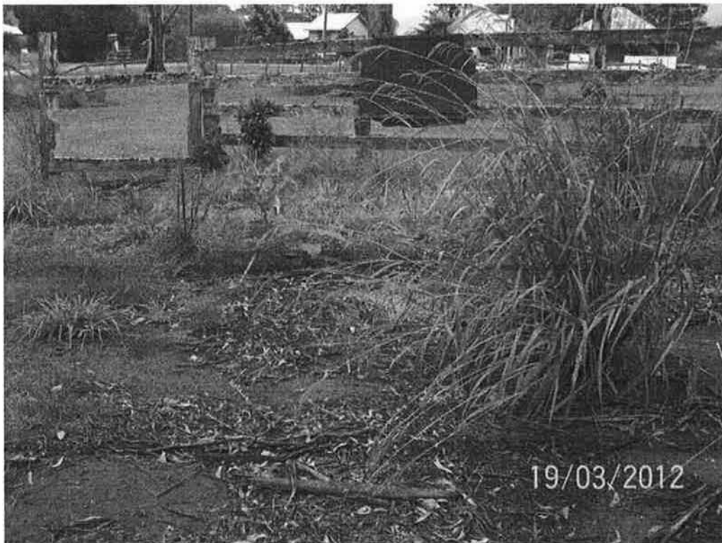
Photo 1 , View of the disused timber stock yards. Soil sample SS01 was collected from the foreground. Samples SS02 and SS03 were collected in a transect parallel to the yards to the north.
